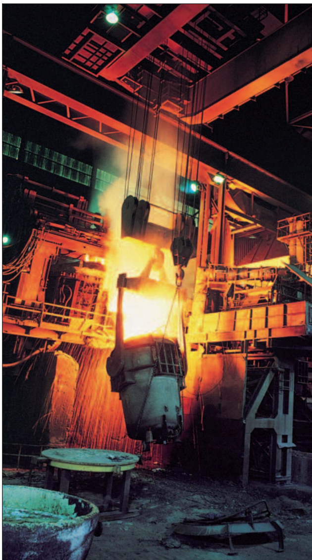
Ladle Crane. Couplings fitted on the input and output of the main hoist and long travel.
